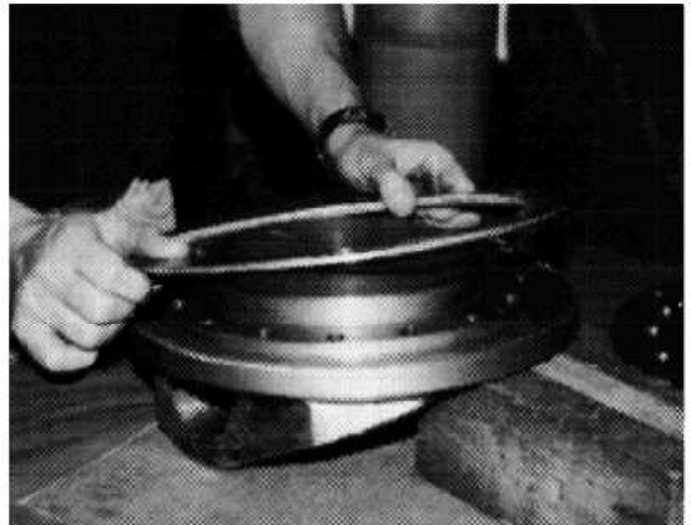
Installing the Gasket
